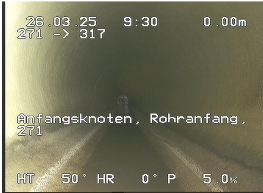
271-317_263.jpg, 00:00:00, 0.00m Anfangsknoten, Rohranfang, 271
