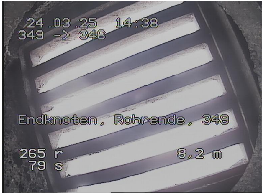
349-346_128.jpg, 00:02:03, 8.20m Endknoten, Rohrende, 349
