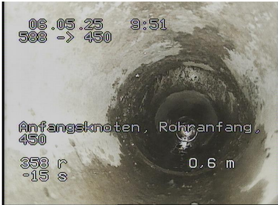
588-450_535.jpg, 00:00:00, 0.00m Anfangsknoten, Rohranfang, 450
