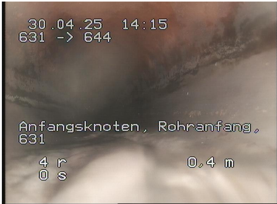
631-644_517.jpg, 00:00:00, 0.00m Anfangsknoten, Rohranfang, 631
