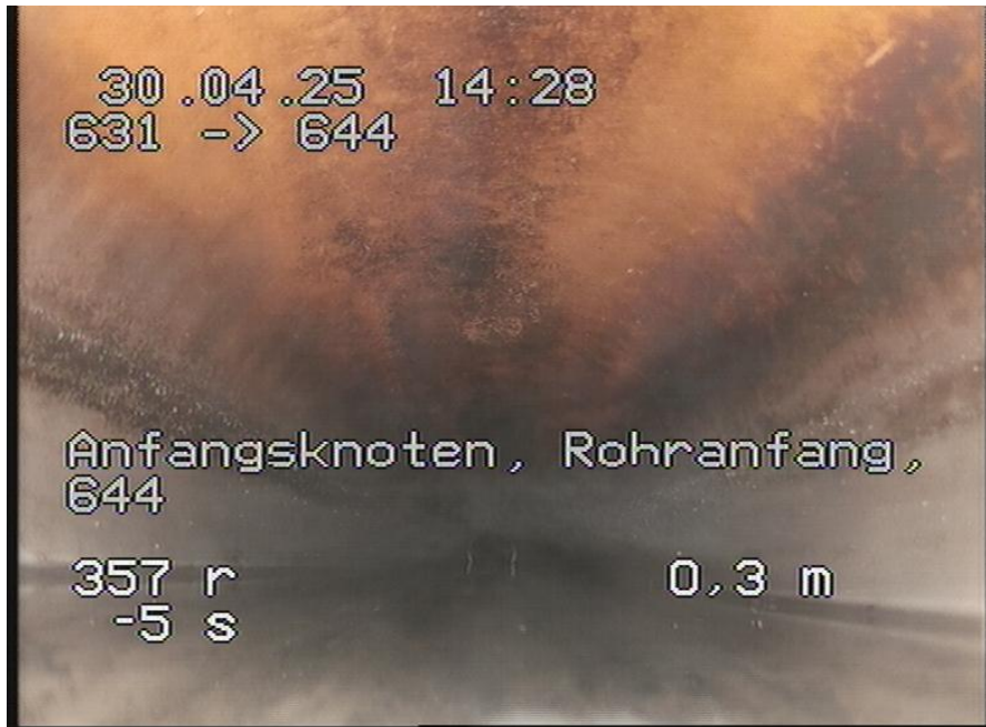
631-644_519.jpg, 00:00:00, 0.00m Anfangsknoten, Rohranfang, 644
